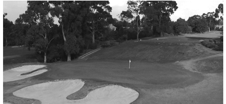
A retaining wall is to be constructed at the rear of the 8th green
